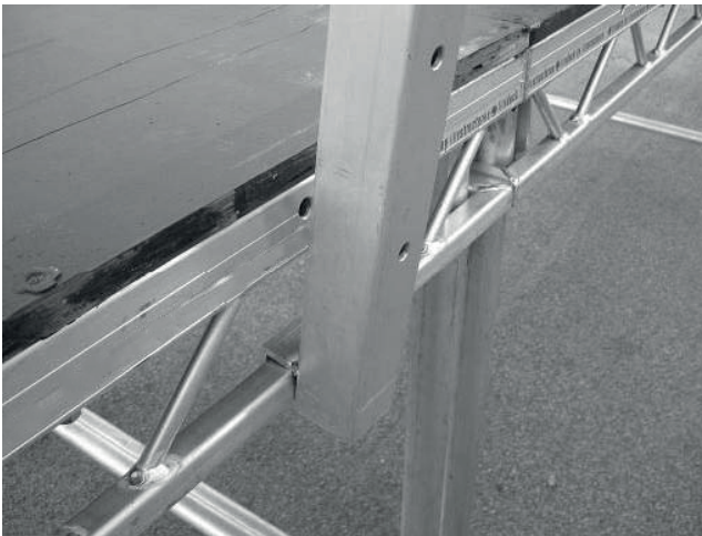
(The holes are lined up and bolts inserted)
