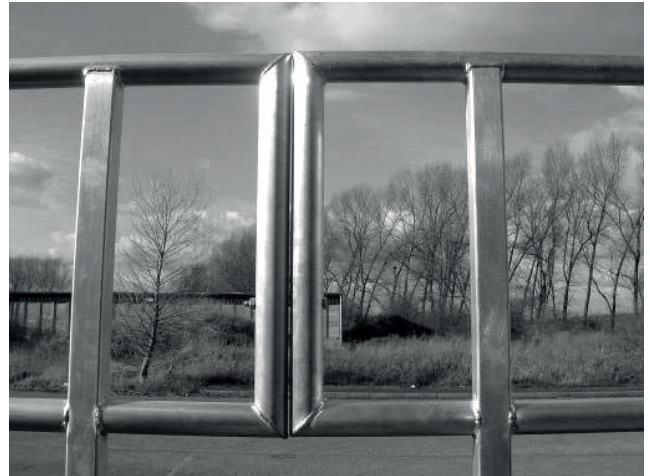
(Bolt is used to join the handrails)
